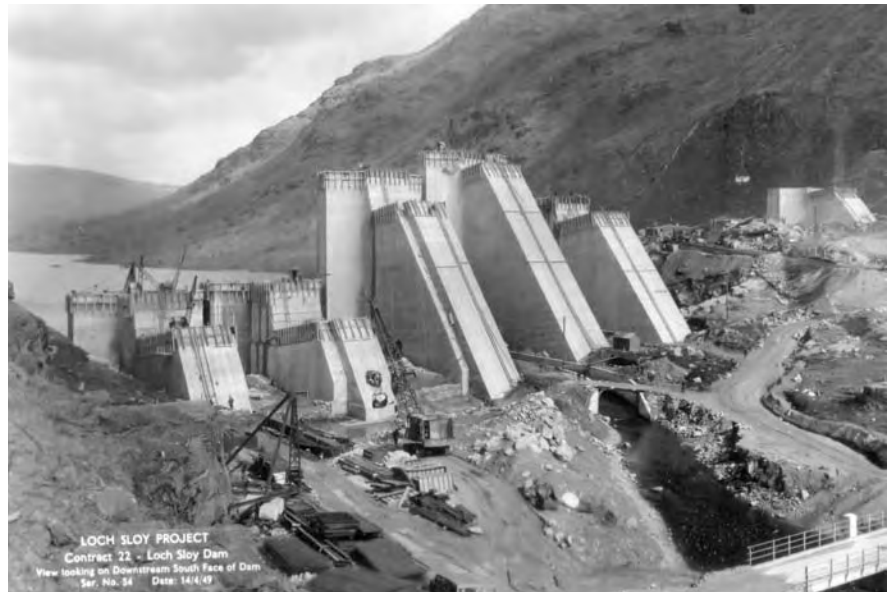
6.2 Downstream face of Sloy dam under construction, 1949, Sloy hydroelectric scheme. © Scottish and Southern Energy
