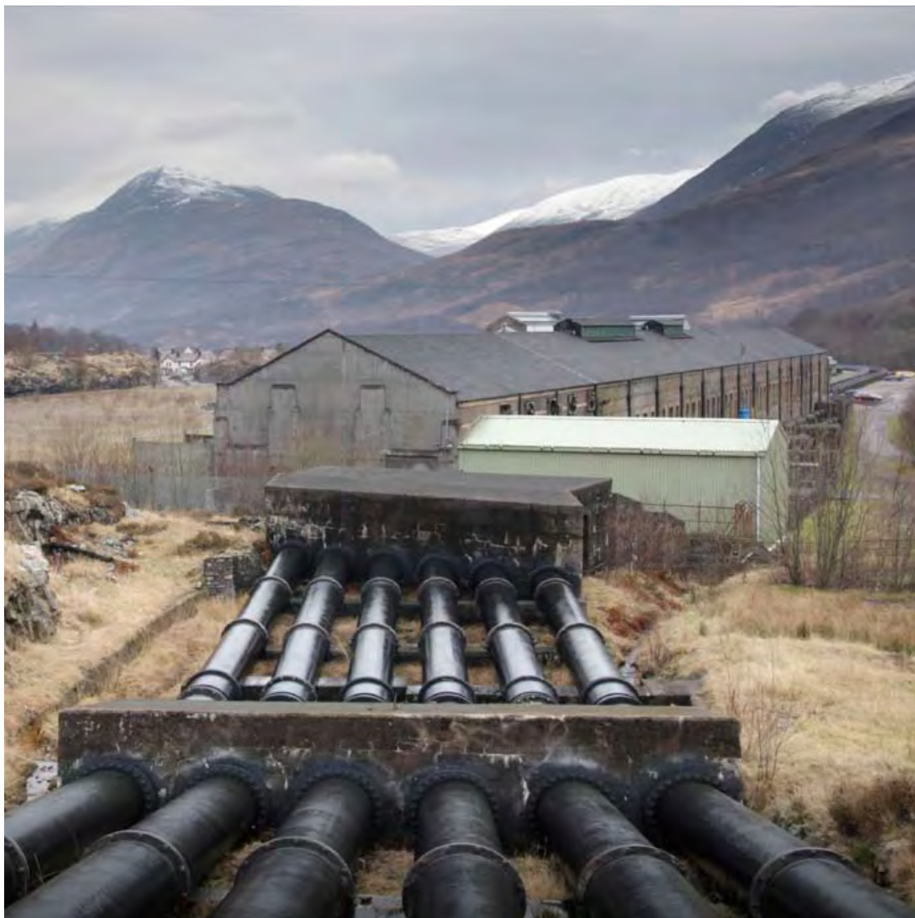
1.7 Kinlochleven power house and penstocks, 1905-1909, Kinlochleven smelter and hydroelectric power scheme.
