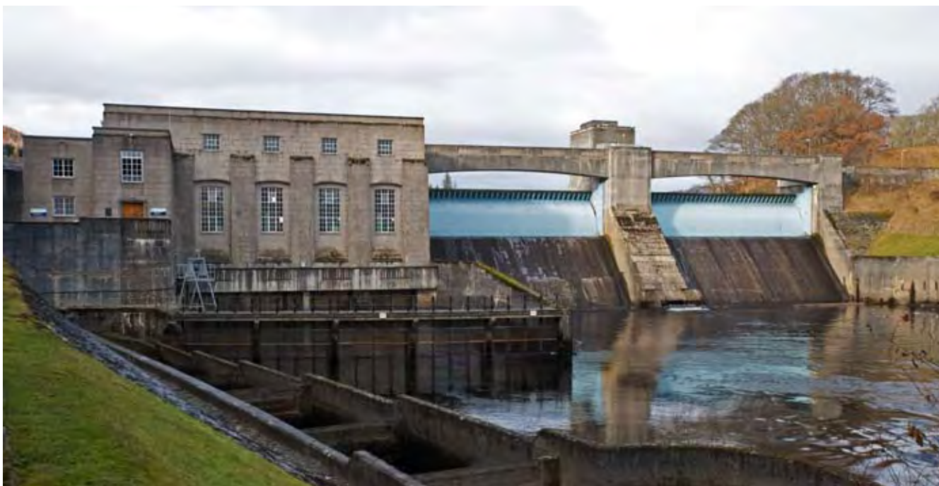
4.6 Pitlochry power station, 1947-1951, Tummel Valley hydroelectric scheme.
