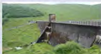
Allt-na-Lairige Dam the first in Western Europe to use pre-stressed concrete for construction.
