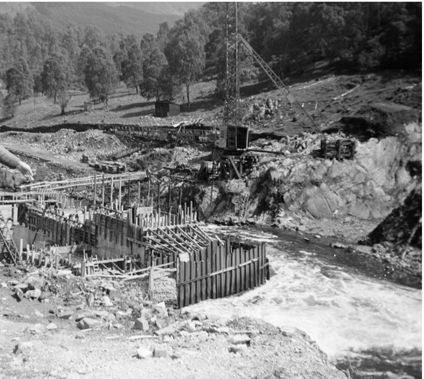
7.5 Construction work during the building of the Tummel Dam, 1947, Tummel Valley hydroelectric scheme. © National Museums Scotland
