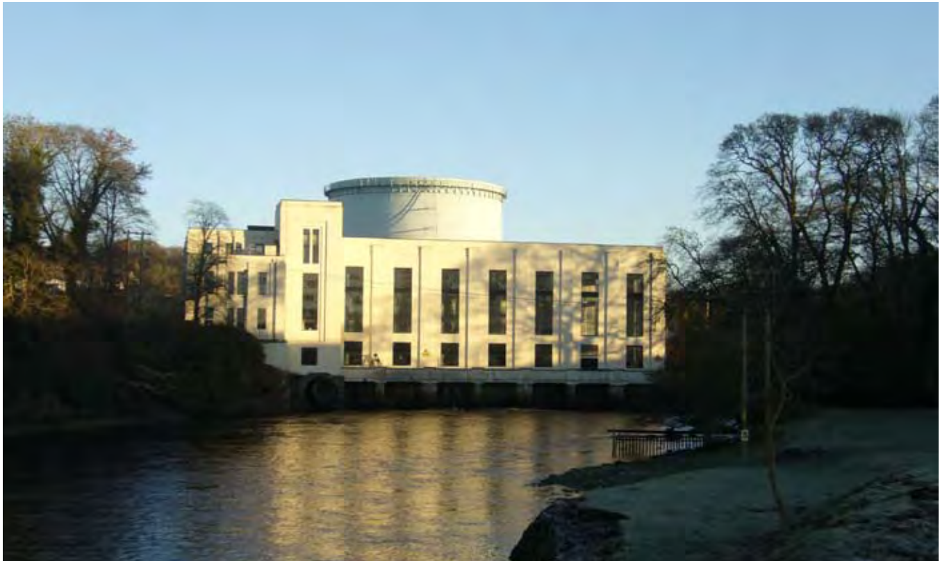
2.6 Tongland power station, 1934, Galloway hydroelectric scheme.
