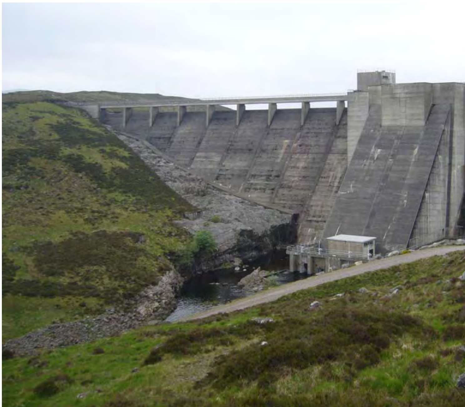
6.7 Orrin dam, 1961, Conon Valley hydroelectric scheme. Orrin dam provides the main water storage for Orrin power station and contains an innovative 4-level fish pass in the large central buttress.
