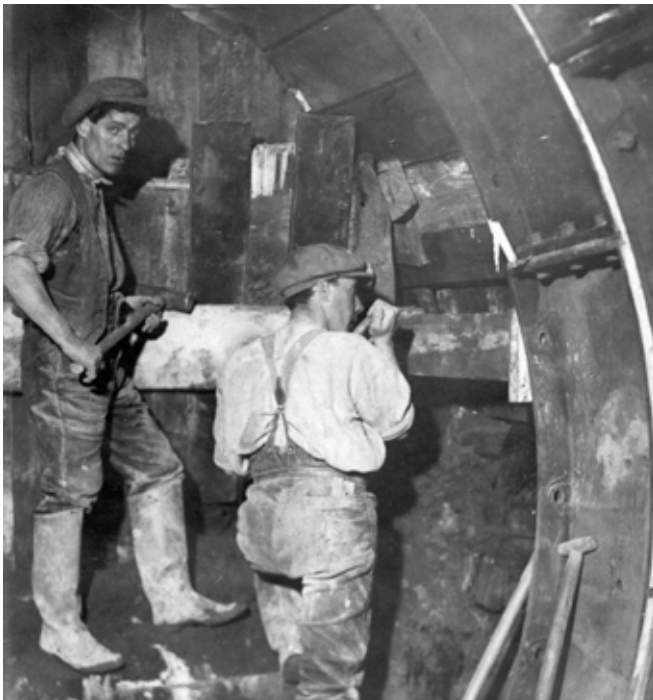
2.4 Workers constructing the tunnel at Bonnington power station, 1926, Falls of Clyde hydroelectric scheme. Crown Copyright: RCAHMS. Licensor www.scran.ac.uk
