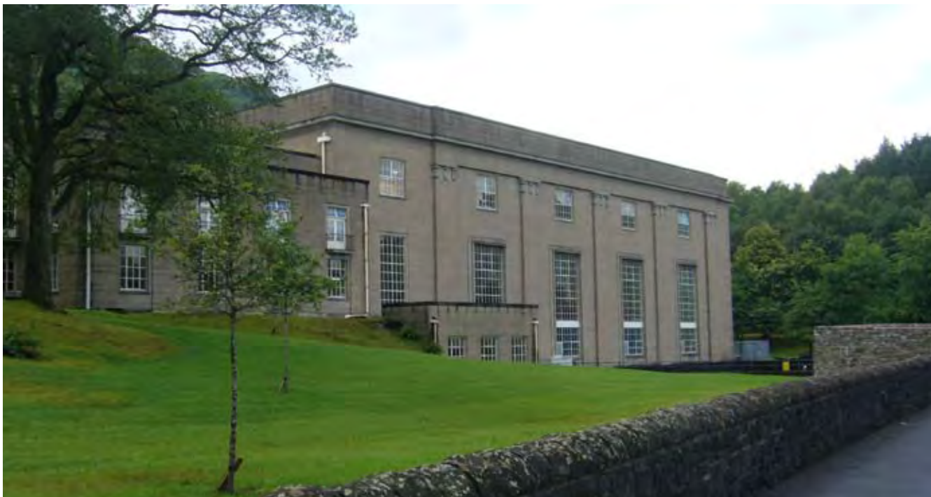
4.3 Sloy power station, 1943-50, Sloy hydroelectric scheme.
