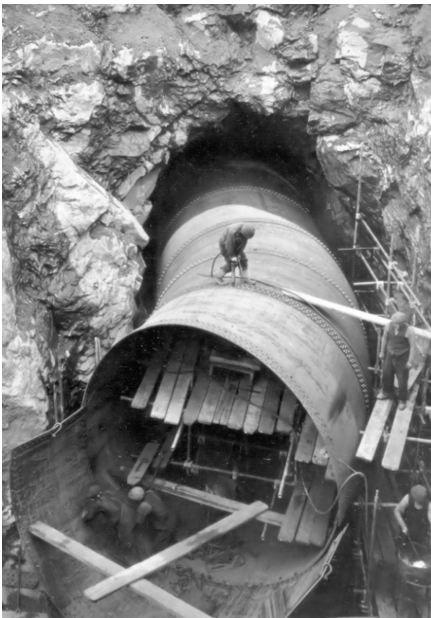
3.6 Construction work on the tunnel at Sloy, 1943-50, Sloy hydroelectric scheme. © Scottish and Southern Energy
