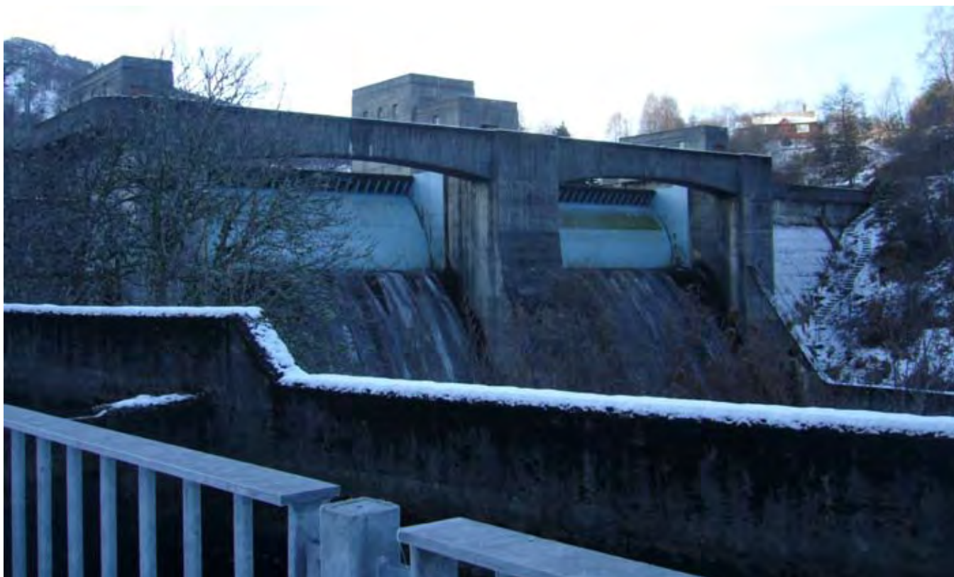
5.8 Clunie dam, 1950, Tummel Valley hydroelectric scheme.
