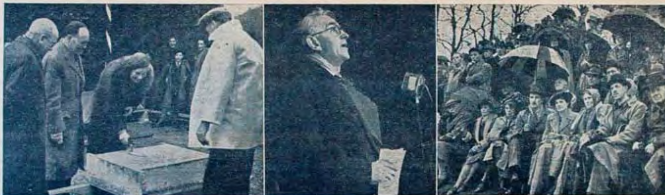
It rained during yesterday's inauguration of the Tummel-Garry scheme at Pitlochry and many of the spectators (right) sheltered under umbrellas. Left, Countess of Airlie lays the foundation stone of the new dam. Centre, Mr Tom Johnston, chairman of the Hydro-Electric Board.
