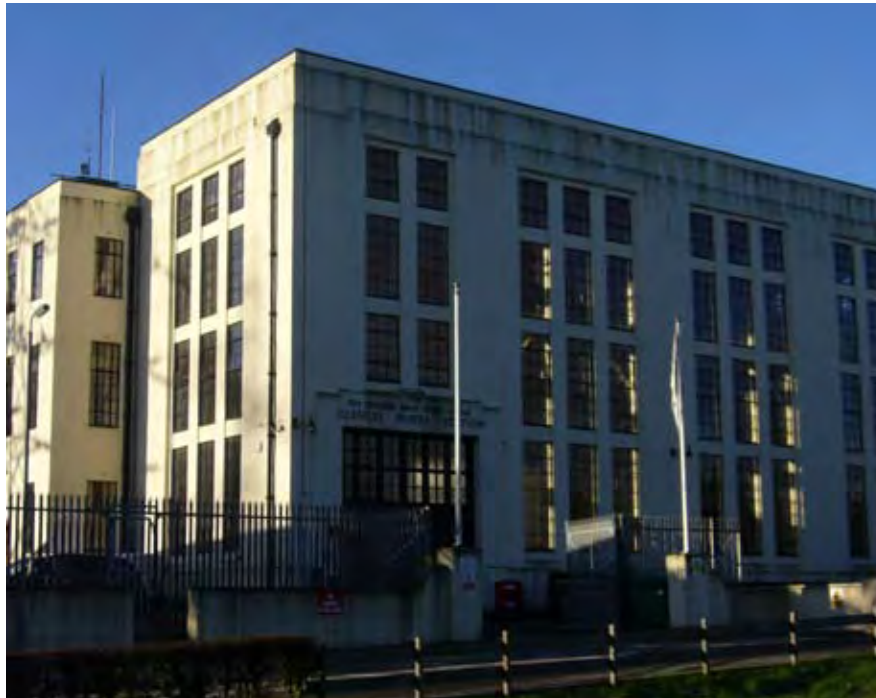
4.4 Glenlee, power station, 1934, Galloway hydroelectric scheme.
