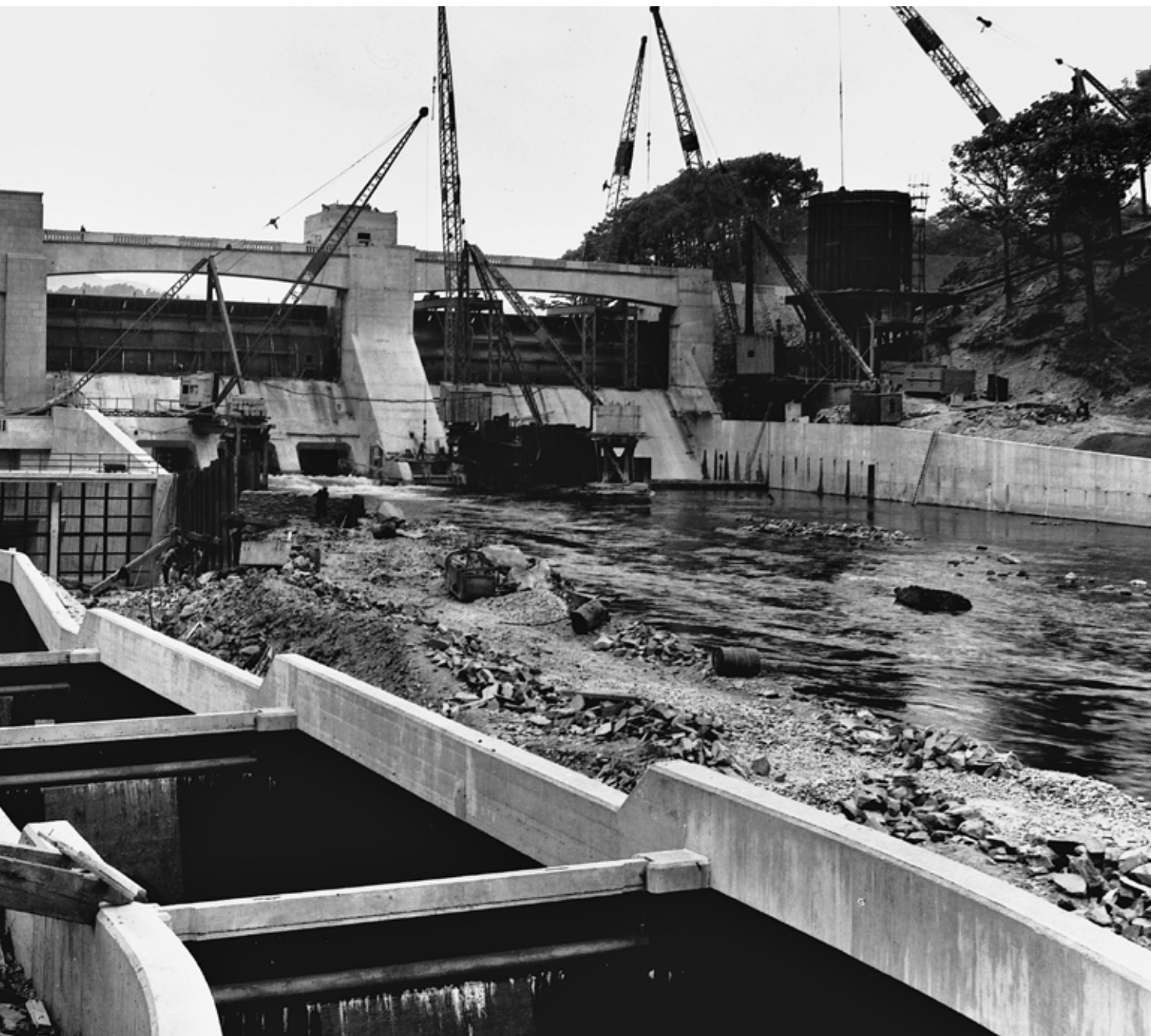
4.5 Pitlochry power station under construction, 1950, Tummel Valley hydroelectric scheme. Crown Copyright: RCAHMS. Licensor www.scran.ac.uk
